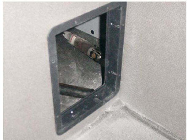
Figure 10 - Return air grill flange installed
